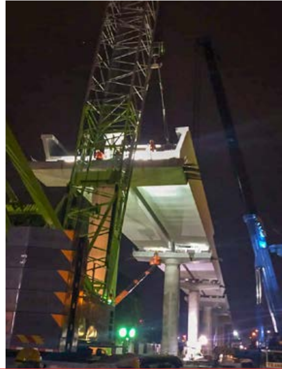
Cargo: U-Trough Girder Dimension: L20-30 m Weight: About 110-185 ton each
